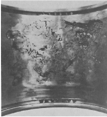
FIGURE 24 Babbitt fatigue in a 7-in (178-mm) diameter turbine bearing. (Westinghouse Electric Corp. Photo originally reproduced in Ref. 8, p.18–19. )
